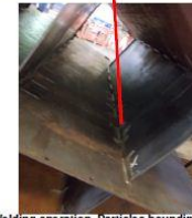
Photo 2- Welding operation. Particles bounding against plates
